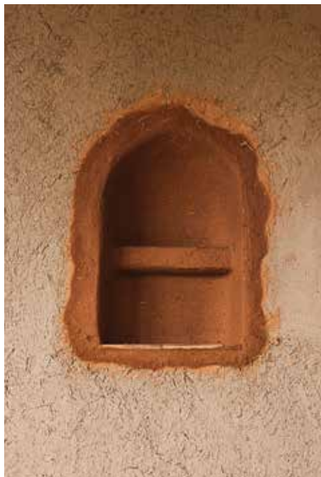
Wall detail inside of James & Alicia's straw bale house on Red Hill
